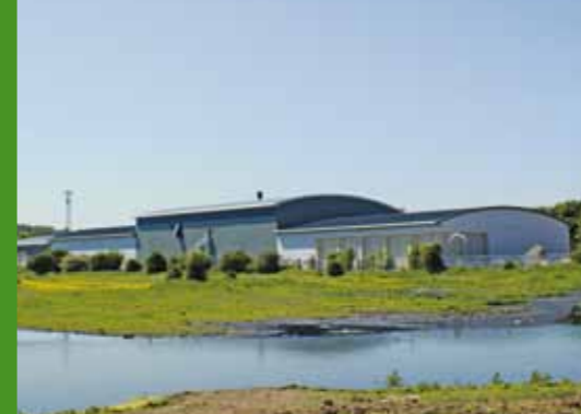
Waste treatment and recycling facility in Newcastle
